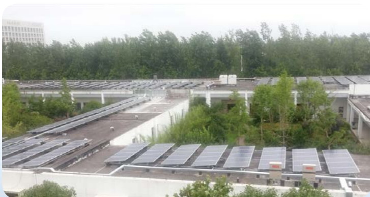
合肥机场屋顶分布式光伏 Distributed Photovoltaic Power Station on the roof of Hefei Airport
