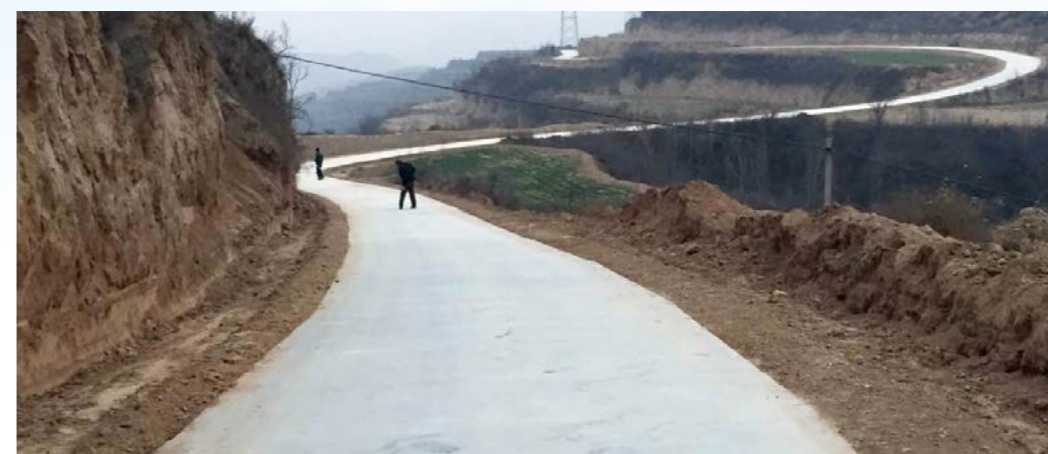
道路硬化后 After road hardening
