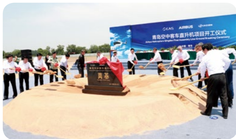
空客 H135 直升机总装线破土动工 Airbus H135 helicopter assembly line broke ground
