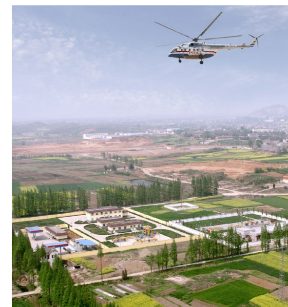
执行西气东输管线巡查任务 Performing the patrolling inspection of the West-East Gas Pipelines
